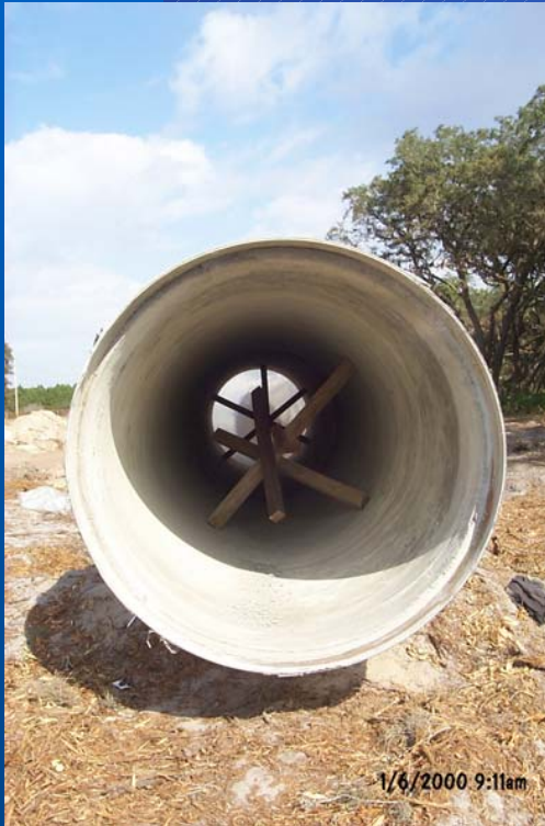
Water transmission pipe
